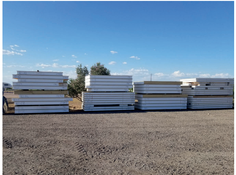
SIPs (Structural Insulated Panels) for the walls and ceiling of the 6-bedroom Bill & Lucille Sapp lodge.
